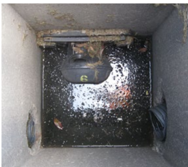
With flow rates starting at 2 LPS/32 GPM, Tempest units are mounted over existing sewer inlets to restrict flow and prevent debris from entering the sewer system.
