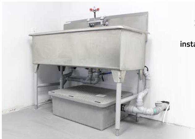
**25 GPM Endura® Lo-PRO Interceptor is able to be installed under bakery's sink with less allowance.**
