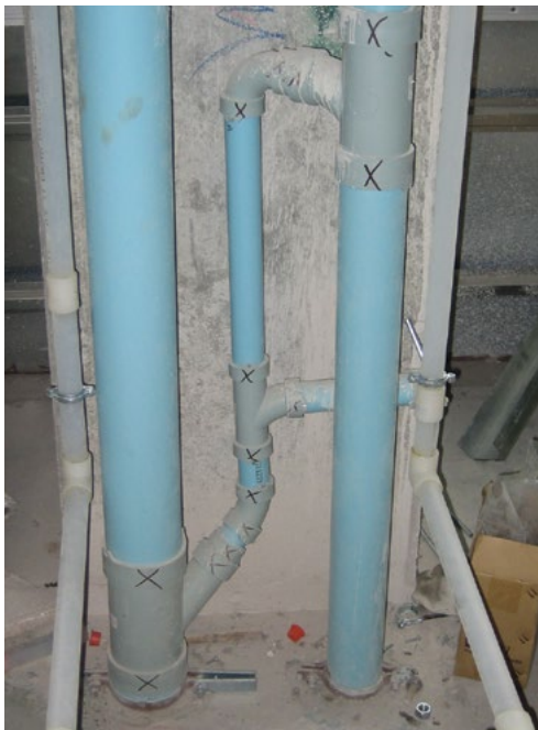
IPEX Labline® & Enpure™ systems being installed
