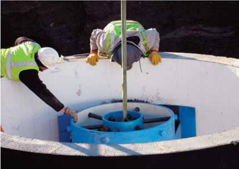
*The easy-to-install Vortex Flow Insert was installed in the Salt Valley 14-foot deep manhole in less than two hours, accommodating a drop in elevation.*
