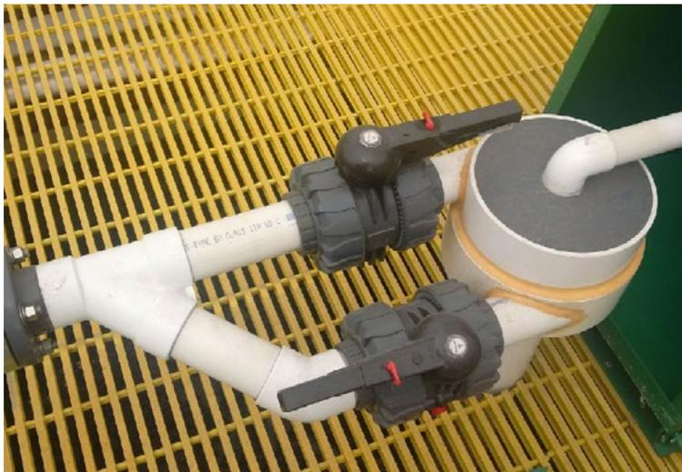
Doug Borrill, Senior Utilities Specialist with the District of Barriere, British Columbia, saw the potential for the Vortex Force to solve a difficult problem at a sewage intake tank. During low flow periods the detention time in the tank would grow, and the sewage would become anaerobic, generating H<sub>2</sub>S and other odorous gasses. While chemical injection was initially considered, Doug had read about Vortex technology in a technical publication and decided to try something new.
