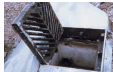
Catch Basin Adjusting Frame
